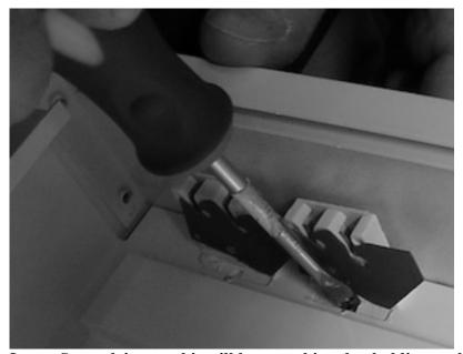
Insert Screwdriver and it will loosen white glue holding socket.
